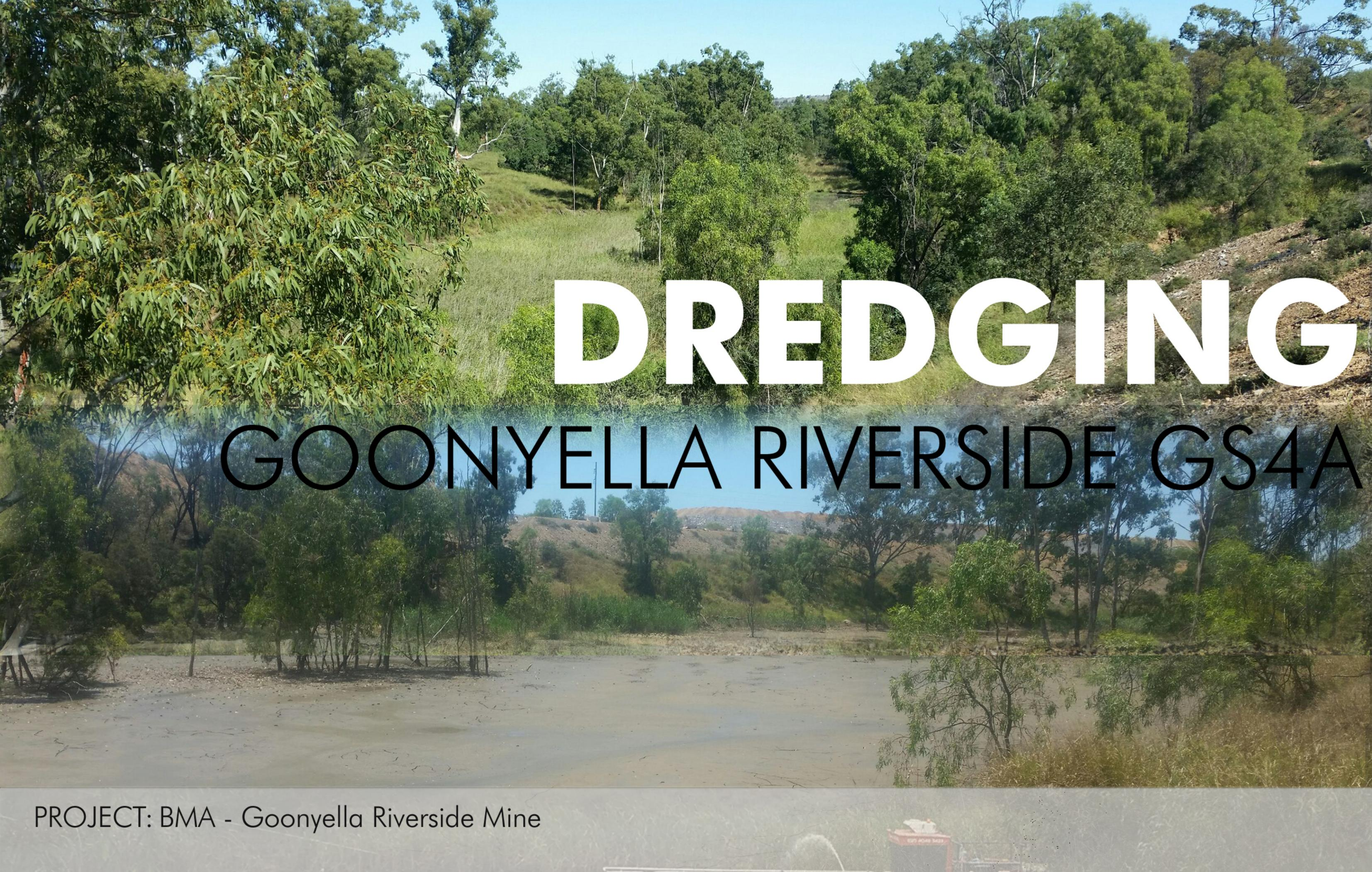
SCOPE: Maxitool Australia was engaged to desilt GS4A which is the final sediment catchment pond for Goonyella Riverside mine before the silt flows into Eureka Creek and off site.
